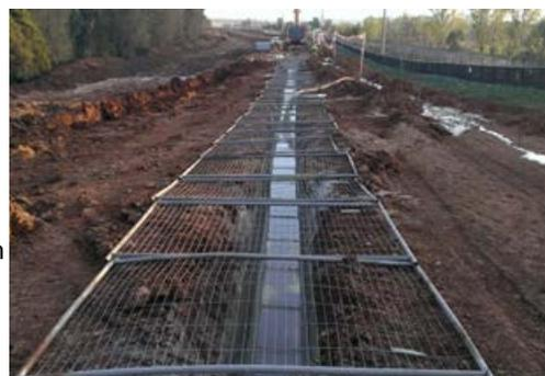
was required to protect the mine from a 1000yr flood event. Due to the presents of alluvial gravel deposits above the bedrock, the cut-off wall was required beneath the flood levee to block off subsurface flow given the increase in water pressure in association to the proposed flood.
