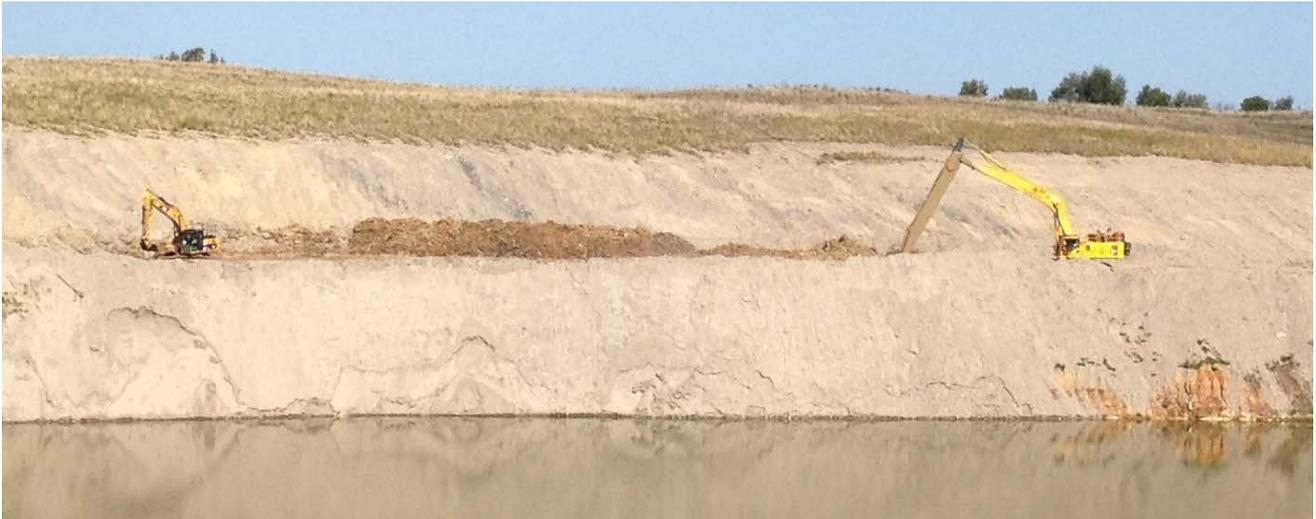
Picture 7: Barrier Wall being excavated through dragline spoil
