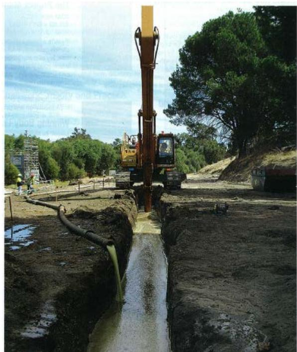
Picture 11: One of two parallel trenches dug to install permeable reactive barriers in Bellevue
