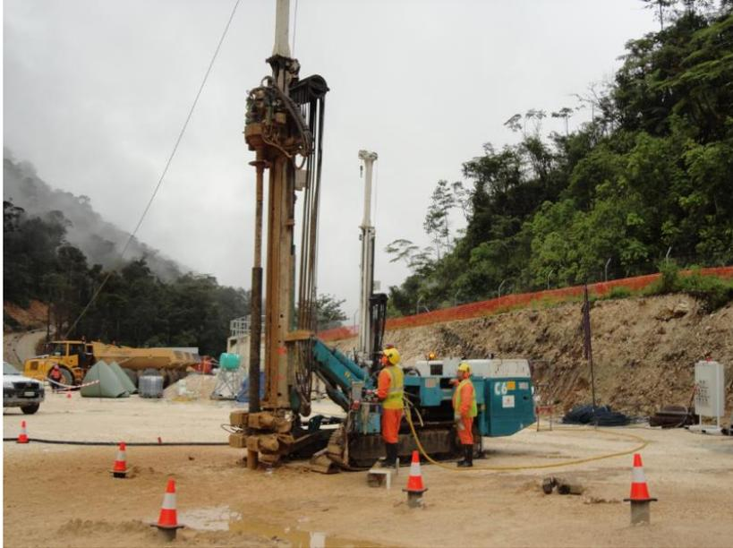
Installation of Ø177.8mm Casing installed in 3m sections
