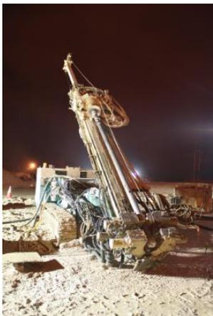
Rig on Nights preparing for next new pile and casing section
