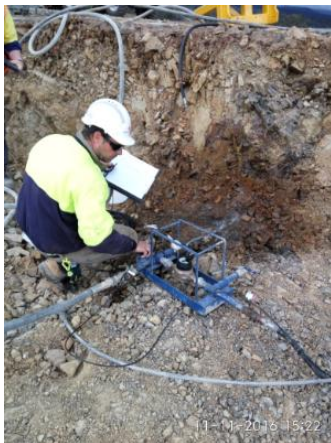
Water Pressure Test
