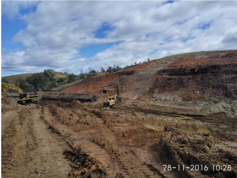
Melrose Dam Foundation drilling and grouting
