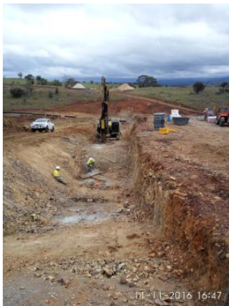
Drilling and Grouting in dam key way
