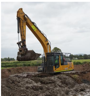
Mixing of virgin soil with bentonite fluid
