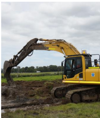
30-tonne excavator during trenching operation
