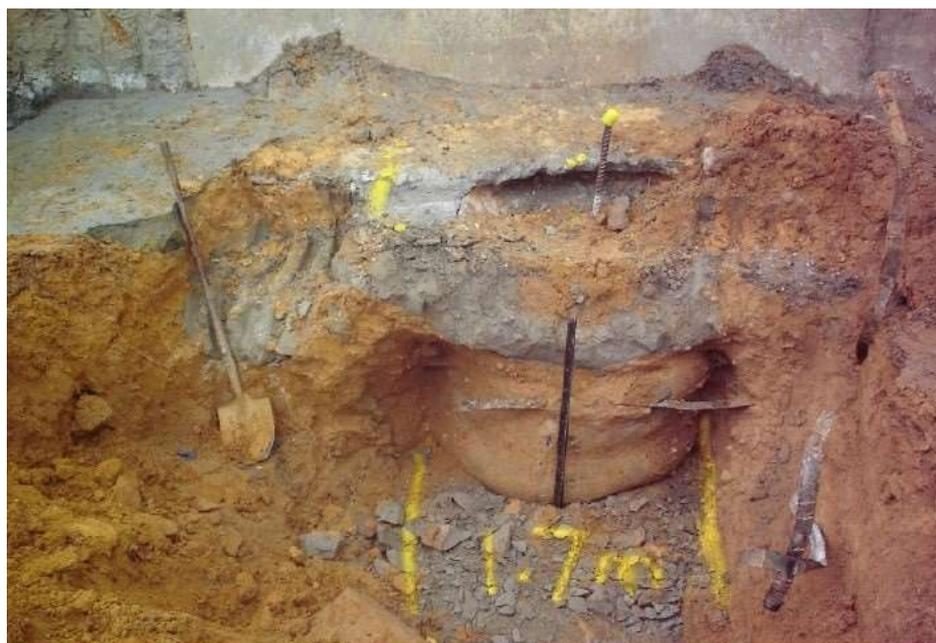
**Figure 9: Trial Column exposed at Beach Road Bridge**
