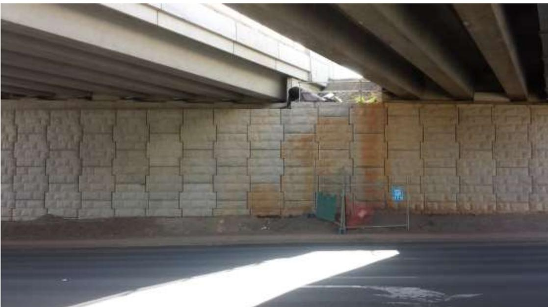
**Figure 16: Sherriffs Rd. Bridge. Bridge abutment duplication finished and bridge deck already installed**
