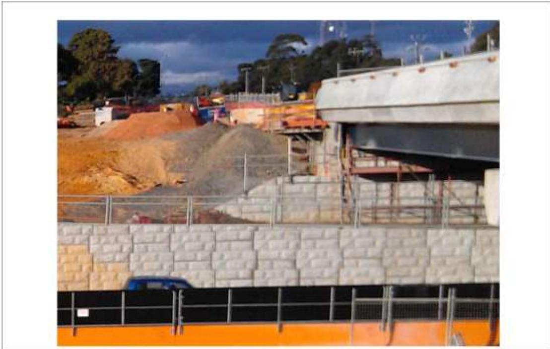
**Figure 15: Beach Rd. Bridge. Bridge abutment duplication finished and bridge deck already installed**
