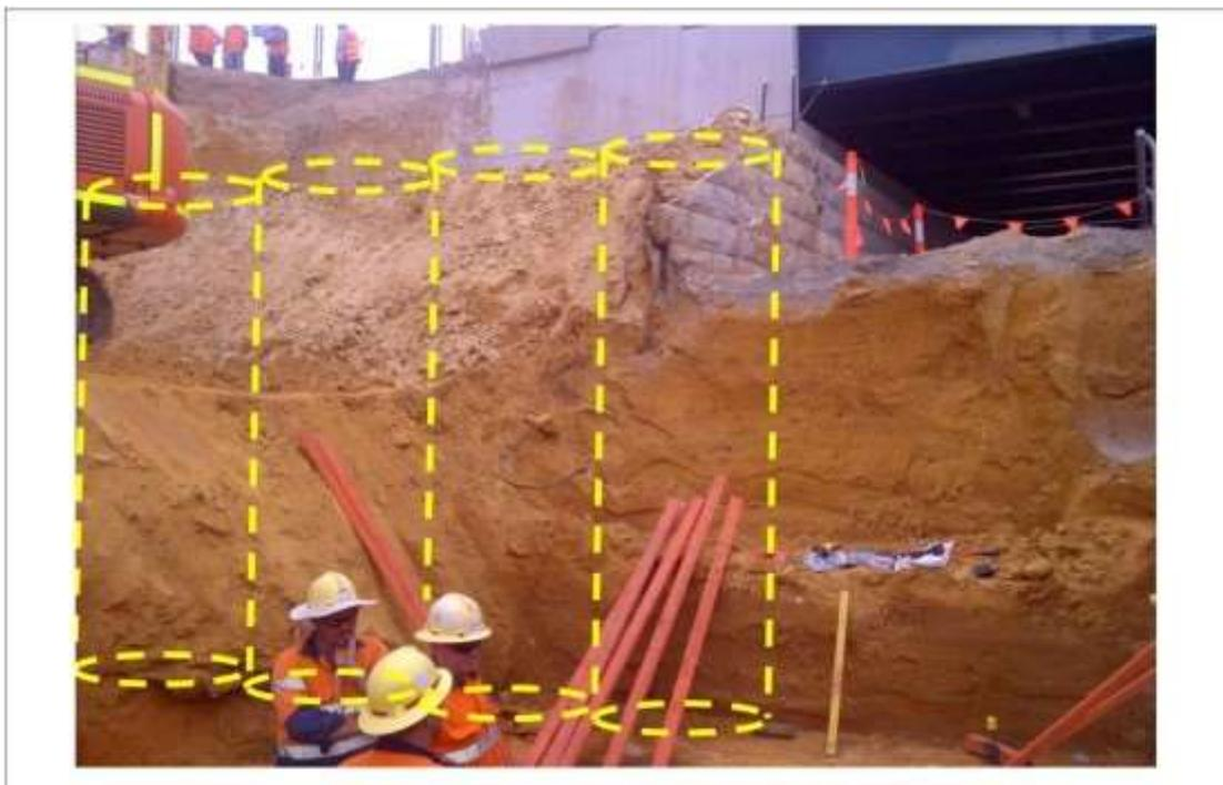
**Figure 11: Beach Rd. Bridge. Concept extent of grouted columns (previously installed)
