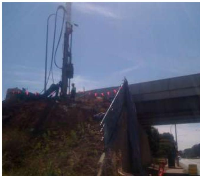
**Figure 10: Installation of JG Columns at Beach Rd prior to wingwall dismantling**
