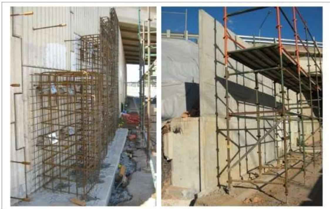
**Figure 5: Cast in situ "new facing" to anchor and conceal nail heads**
