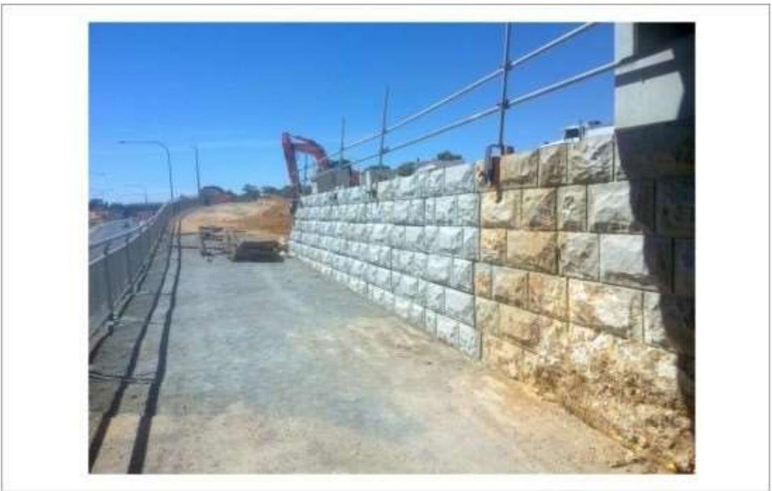
**Figure 14: Beach Rd. Bridge. Duplicated abutment facing following completion of construction**
