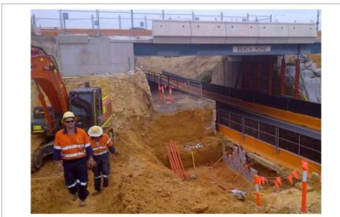
**Figure 12: Beach Rd. Bridge. The installation of jet grouting columns allowed for an almost vertical excavation profile**
