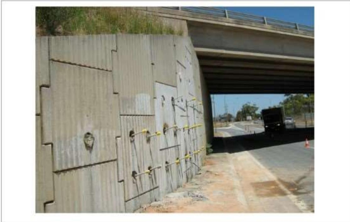
**Figure 4: Typical soil nailing strengthening operations**
