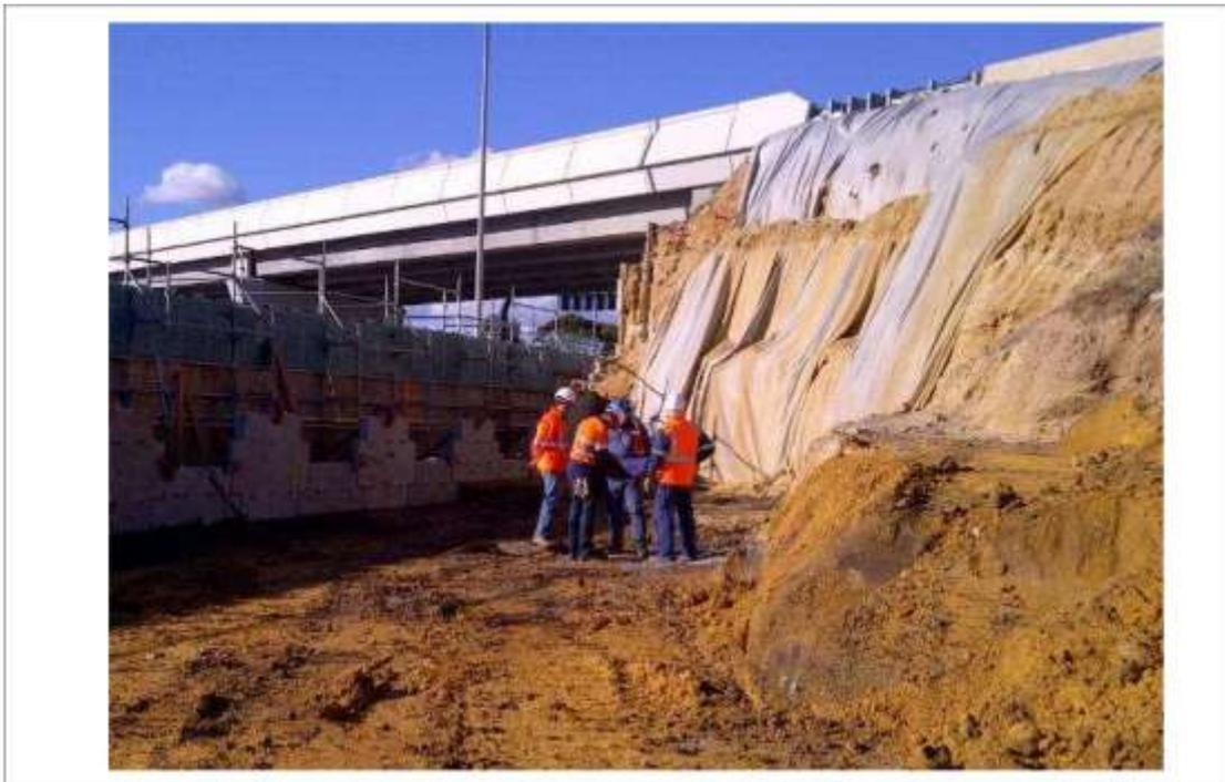
**Figure 13: Beach Rd. Bridge. The installation of jet grouting columns allowed for a stiffer excavation profile than other solutions**
