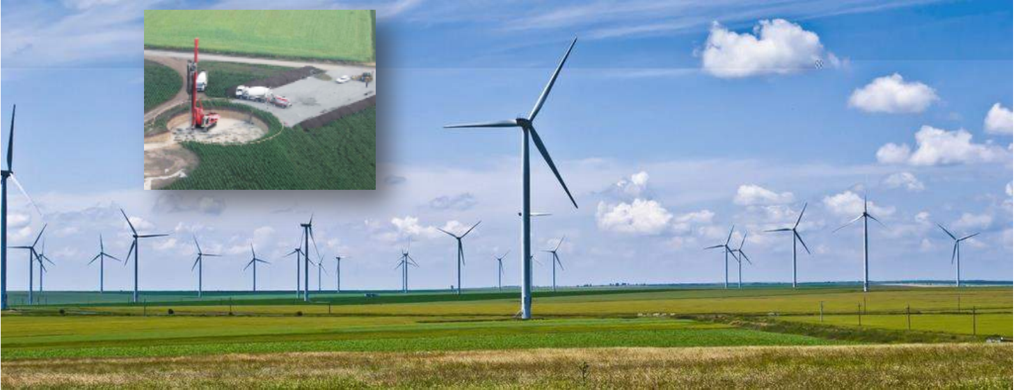
Largest European and world's 9 th largest wind farm: Fântânele-Cogealac Wind Farm
