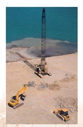
In some cases, the location of the Dynamic Replacement Columns can be pre-excavated. The excavation is then partially backfilled with a "plug" of granular material. This initial plug is then driven into the soft layer by the tamping energy of the weight to the required depth of treatment. This crater is regularly backfilled with additional granular material between each tamping phase.
