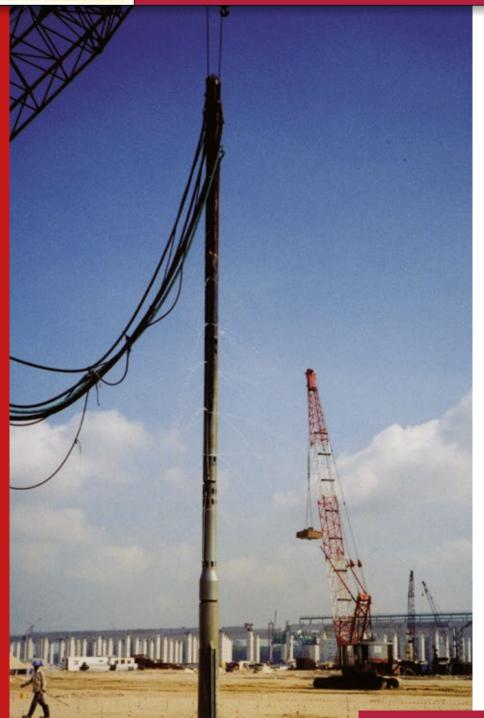
A loose soil or heterogeneous granular backfill can be compacted in depth by the penetration of vibrating probes or vibroflots. The main purpose of vibrocompaction is to densify the in-situ soils by vibration.
